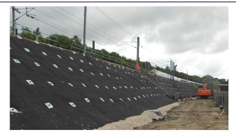
Package 606 was a Design & Construct contract involving stabilisation, earthworks and drainage improvements to embankments and cuttings on 3 separate sites across the North West rail network.
